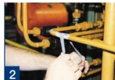
2 remove paint and clean pipe
