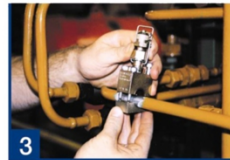
3 clamp SC onto pipe
